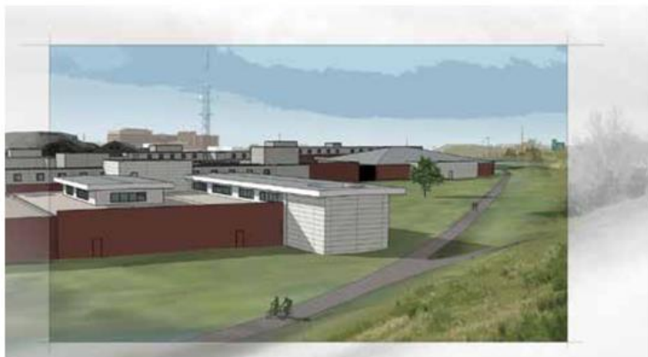
Construction began on an expansion to the 43,000-square-foot Tulsa County Jail in May after an April groundbreaking ceremony.
