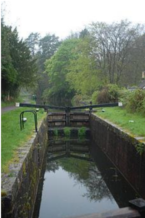
Figure G-13 - Canal Conveyance
