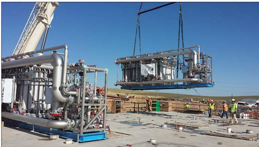
Ceramic membrane filter 2 being installed at Rueter-Hess Water Treatment Plant
