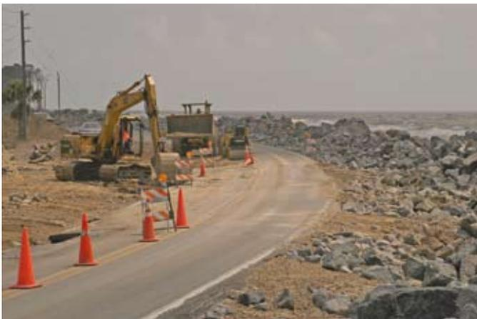
**Cape San Bais, Gulf County, FL, 8-31-05: Crews make emergency repairs to this damaged road after Hurricane Katrina washed away a rock sea wall that was built to protect it. Credit: Marvin Nauman/FEMA**
