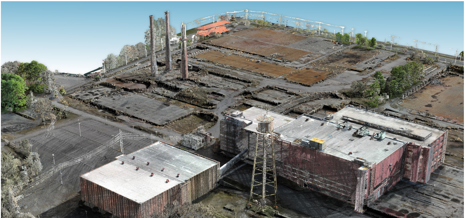
This colorized point cloud data of the historic mill site redevelopment was acquired using the TrueView615 sensor on the Inspired Flight IF1200 sUAS.
