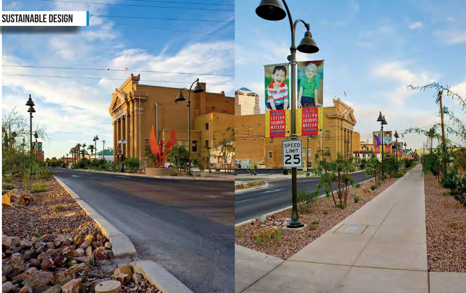
Stantec transportation green infrastructure/low-impact development application on Scott Avenue Roadway, City of Tucson, Ariz. Photos: Courtesy of Stantec
