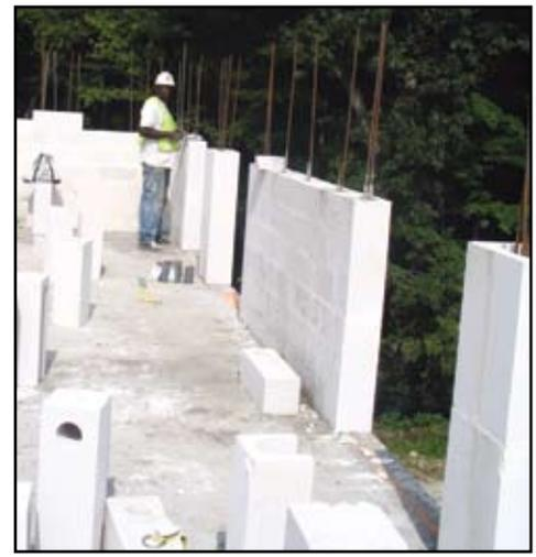
*Installation of AAC reinforced block walls at State University of New York at Stony Brook.*
