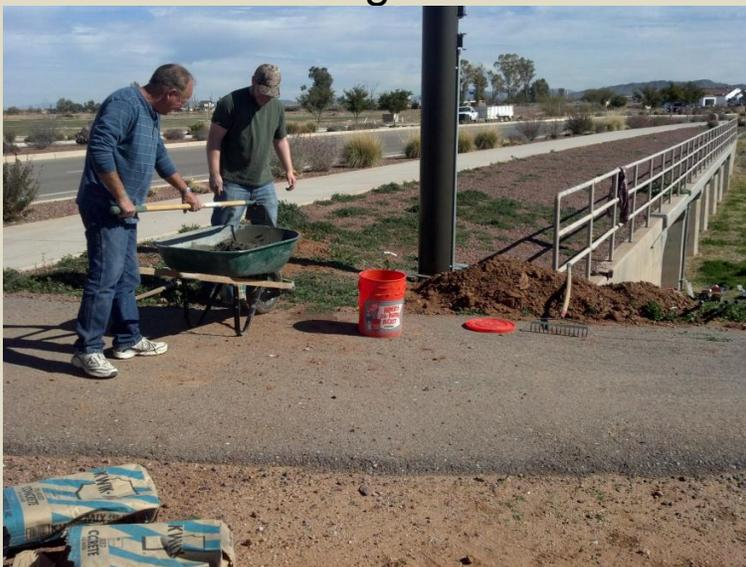
Tyler Azeltine (right) of JE Fuller Hydrology helps Lonnie Sanders of the Pinal County Flood Control District install a new ALERT stream stage station near Red Rock, Arizona.
