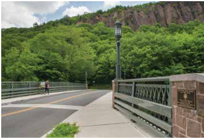
The rehabilitation replicated the ornamental pedestrian rail system and added decorative lighting.
