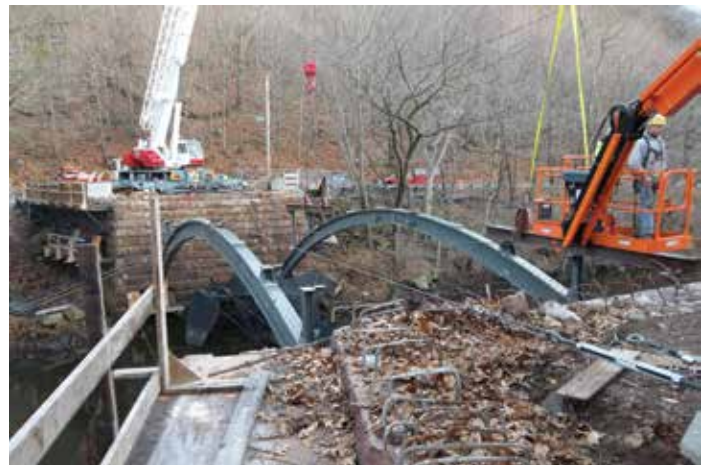
Construction views showing erection of rehabilitated steel arches.
