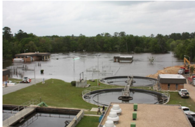
Figure E.2. Withlacoochee River Wastewater Treatment Plant, Valdosta, GA. LiDAR is vital for proper locating of water and wastewater facilities, or, in this case, the relocation of the plant. Image courtesy of the Georgia Geospatial Advisory Council (GGAC).
